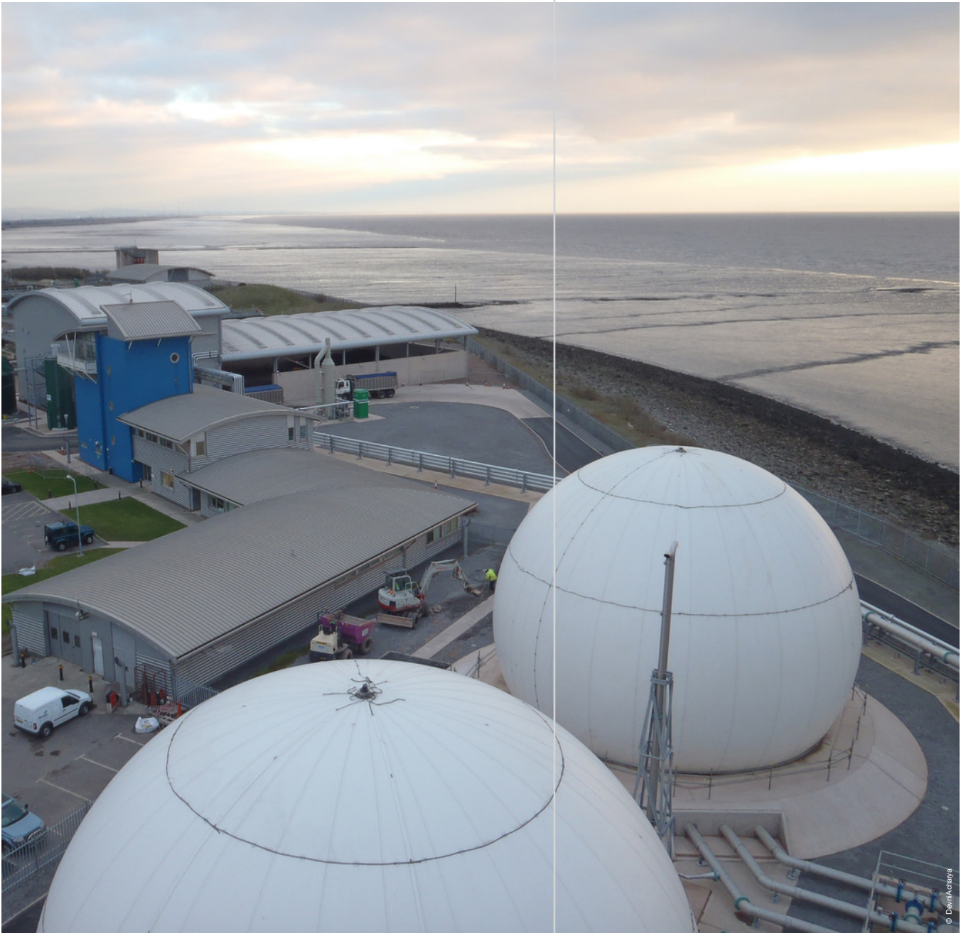
Right: Anaerobic Digesters, Cardiff WWTW
